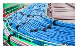
Overly dense rack system cabling is difficult to manage and wastes valuable space (above).
